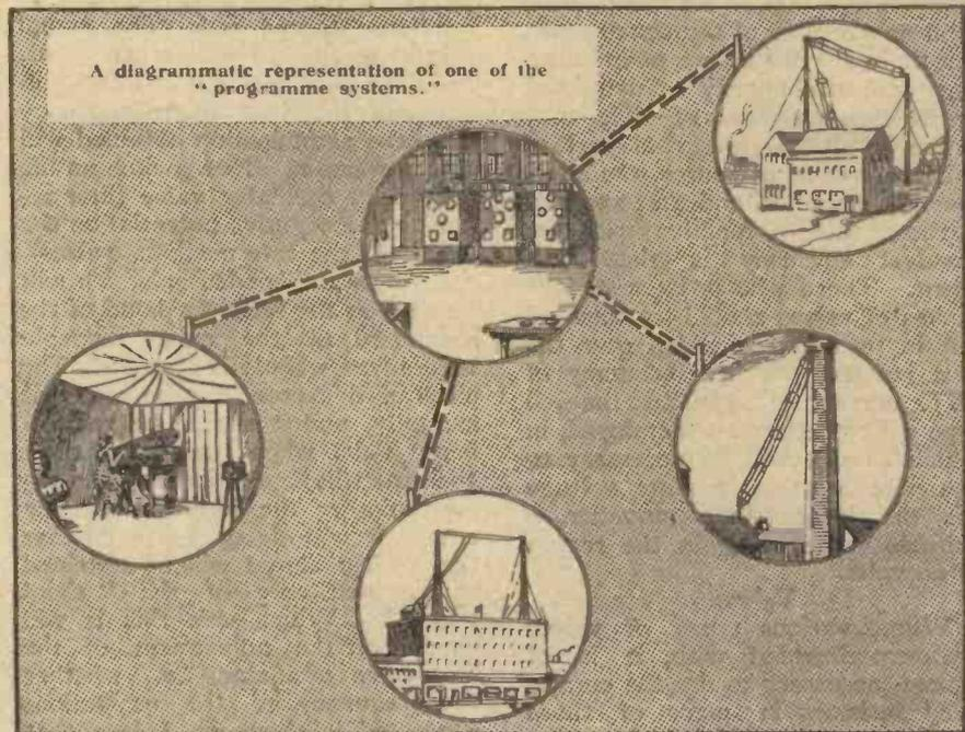
In the scheme suggested each of the three programmes would be distributed by "Wired Wireless" to the various transmitting stations.
