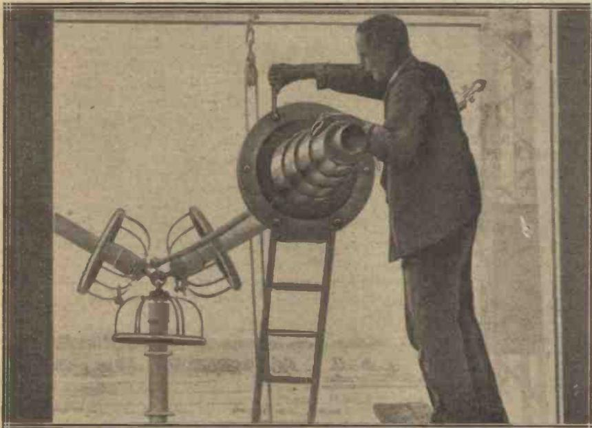
Fitting the giant leading-in insulator to the window through which the aerial lead passes.
