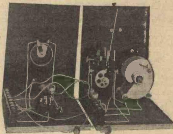
the tuner panel A, the valve detector panel B, and the first-stage L.F. amplifier panel C. This arrangement may of course be employed with or without reaction, and should give full loud-speaker strength on local signals.
