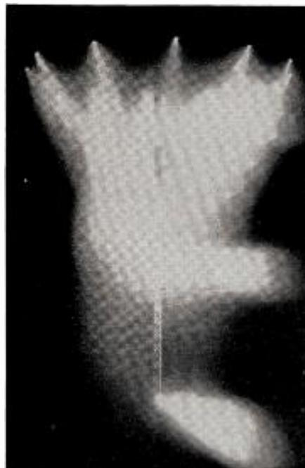
THIS is the scene that an airplane pilot will see at night if current experiments by WHAS Louisville for substituting "area" lighting for structure lighting work out. It is one of the first experiments to define a radio or tv tower and guy wires to improve the visibility of tall towers for pilots. WHAS-TV has proposed a 2,000-ft. tower; this is how it will be lighted if current tests on the WHAS tower prove out.
