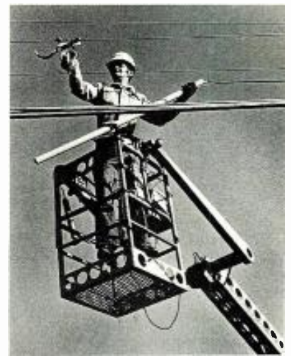
Hang it up. A Cablecom-General technician strings the Joplin fiber-optic cable.
